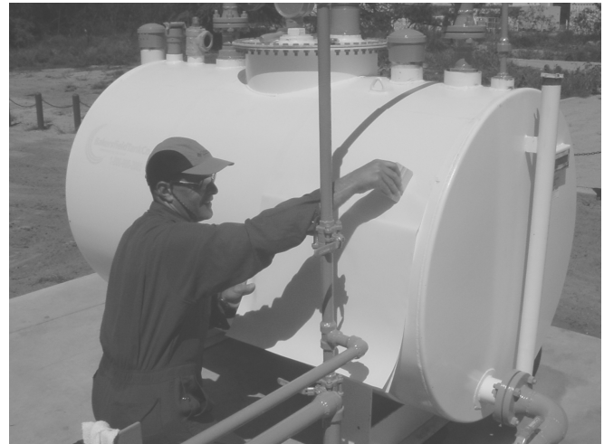
Figure 9. Application of appliqué on tank at Pacific Missile Range Facility.
