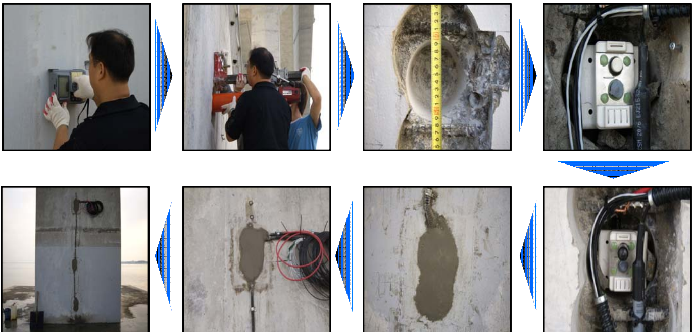
FIGURE 4. Installation of an RCCM on a Bridge Pier.
