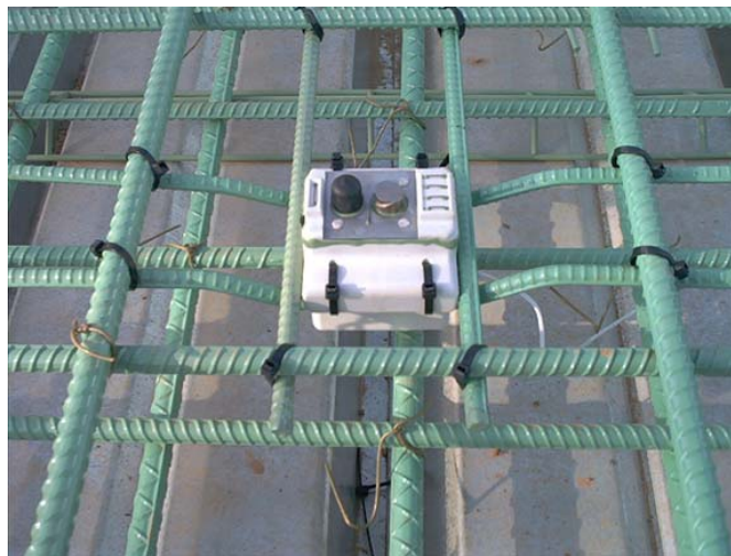
FIGURE 1. RCCM Installed on a Rebar Grid.
